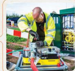
Fibre-optic cable is blown into multi-duct
