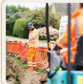
Excavation of trench for duct
