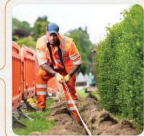
Trench reinstated leaving minimal 'scarring' to the surface (in some cases, temporary reinstatement is required until the network is completed)
